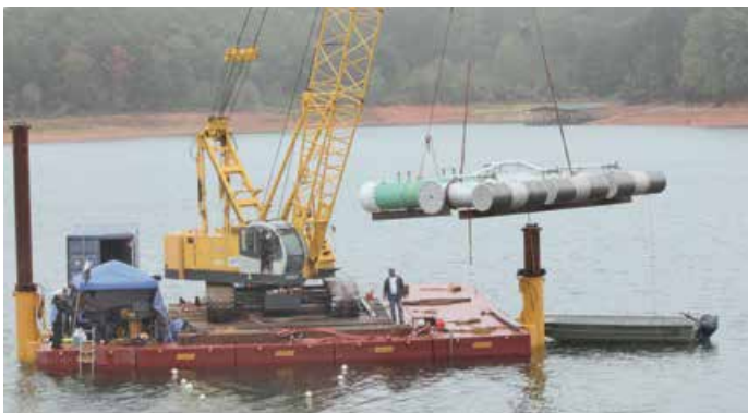
Johnson Offshore Intake Systems™ (JOIS™) Installation
