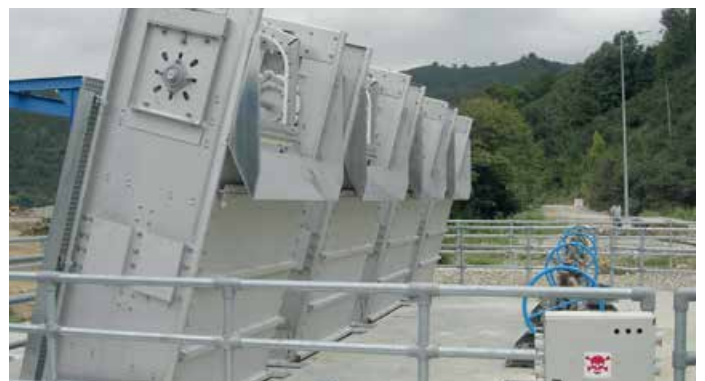
Geiger® High-Capacity Revolving Chain Screen
