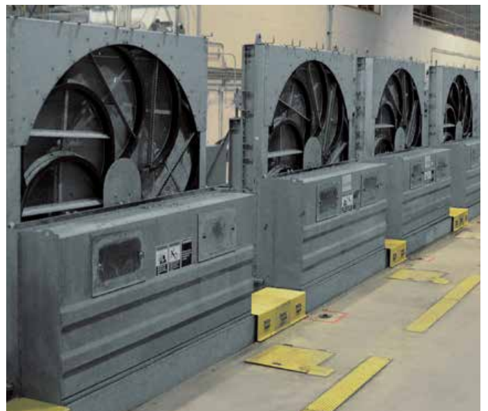
DC Cook Nuclear Power Plant, USA
