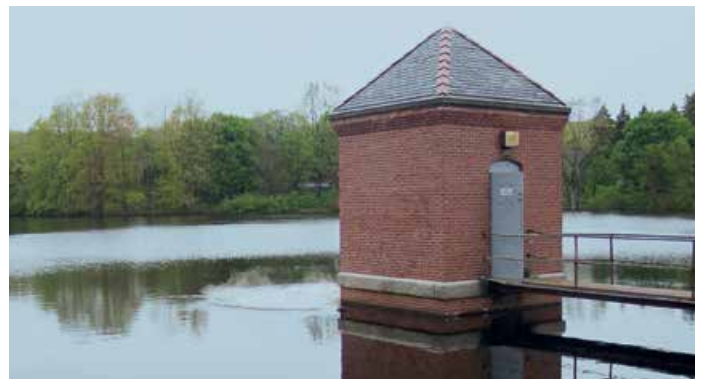
Hydroburst™ with Surface Blast
