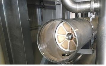
Figure 2 Wastewater tank with BIO-CEL® L-1 modules installed
