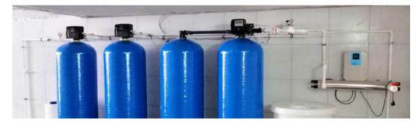
In a water treatment system, filters essential for improving effectiveness of subsequent stages, when correctly selected, reduces load of successive systems, improves efficiency of the device and decreases costs.
