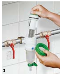
3. Extract the flow diverter with the cartridge from the filter body.
