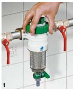
1. Shut off the water at the both sides of the filter
