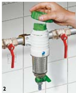
2. Turn the ring nut counter-clockwise until it is released.
