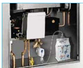
Installation of MiniDUE cod. PM006 with remote Kit.
