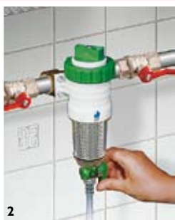
2. Open the discharge tap for few seconds 3. Close the tap and switch the knob to the original position.
