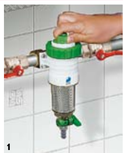
1. Change the water in-take by switching the knob from IN DX to IN SX or vice-versa.
