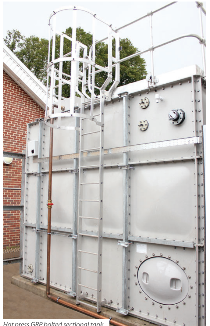
Hot press GRP bolted sectional tank
