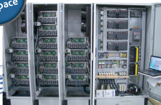
Situation after installing Nedap UV lamp drivers
