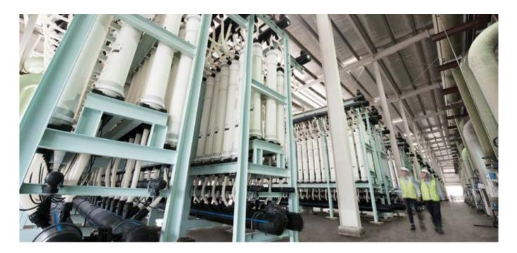
Developed, tested and fabricated in Singapore, Kristal<sup>®</sup> polymeric ultrafiltration (UF) hollow fibre membrane has been one of Hyflux's main product lines since its launch in 1999. Hyflux's technological innovations have taken Kristal<sup>®</sup> ultrafiltration technology to the next level. Today, Kristal<sup>®</sup> membranes are used in a wide range of applications in water treatment and wastewater recycling.
