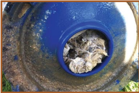
Ragged pump before installation of DERAGGER II ® anti-ragging device.
