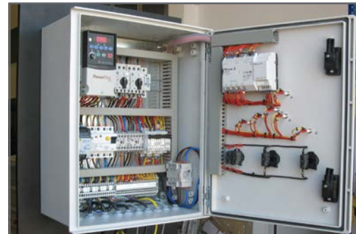
VSD for automatic powder feed flow regulation
