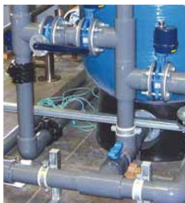
Maric valves control backwash flow rate in a media filter
