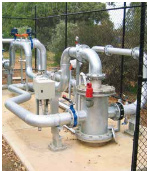
Submersible pump installation
