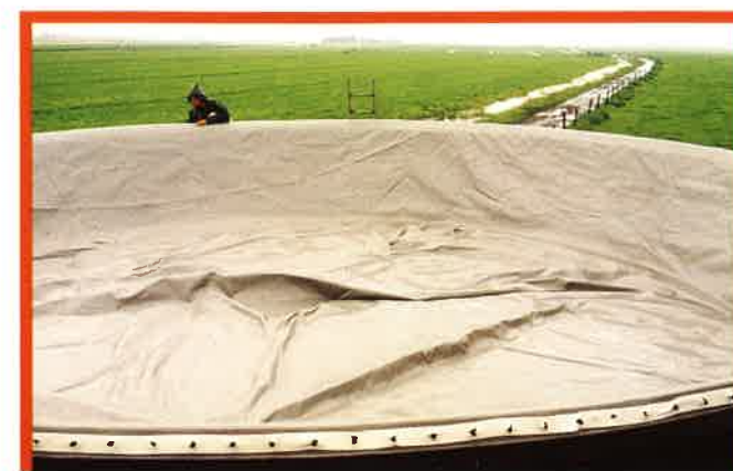
"Zeppelin"-shape membrane gas holder for installation in support frame
