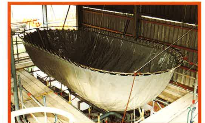
"Zeppelin"-shape membrane gas holder for installation in support frame
